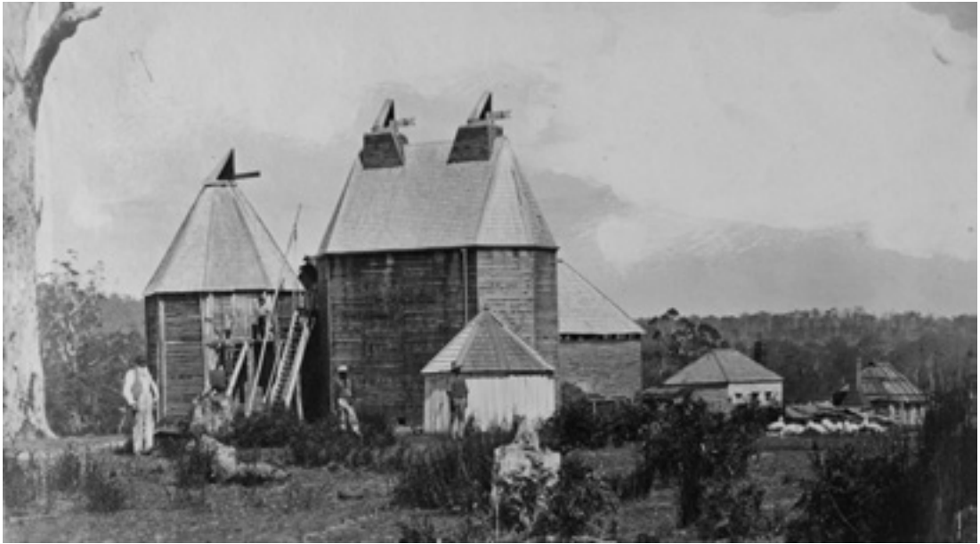
Figure 9. The hops kiln at Coranderrk (c.1870s). Source: Museum Victoria (XP1931).
